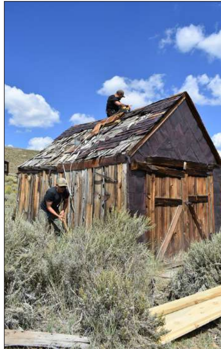
Park employees stabilize a Bodie building in 2019.
