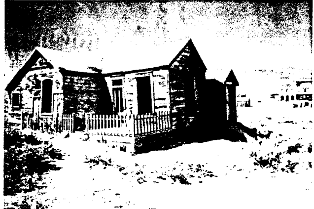
Fouke House after stabilization was completed
