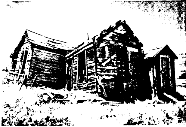
Fouke House before work began
