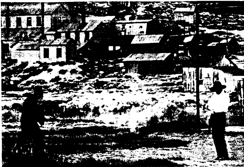
A shootout in front of the Wheaton and Hollis Hotel between Maintenance Worker I Charles Spiller and Ranger Mark Pupich
