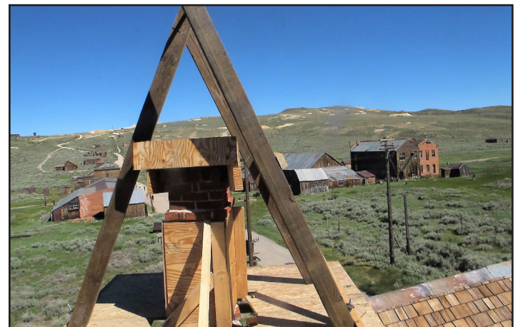
To repair the J.S. Cain house chimney, workers built a platform and clamped the chimney down with compression straps. They then put on an A-frame, lifted the chimney a couple of inches and put it back square. Photo by Paul Serna-Garcia
