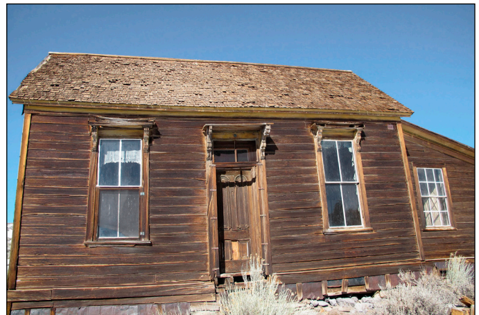
The Kirkwood house (above and below) will benefit from roof repairs, siding re-attachment, and interior stabilization and repairs. Foundation members can take pride in the restoration work that will benefit all of Bodie's visitors.
