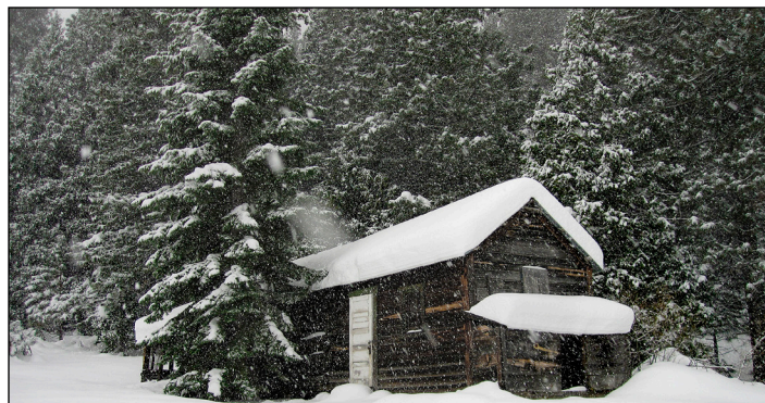
A cabin sits on the site of Alvin Grover's Hot Springs Hotel, which burned down in 1919. The structure was later used as a summer cabin for a ranch family and is now used as occasional living quarters for park personnel.
