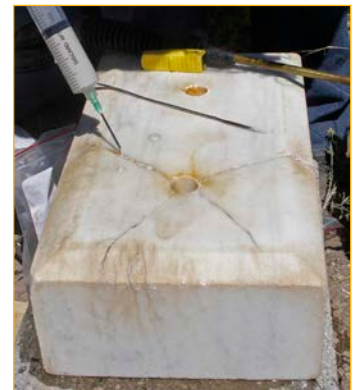
Jennifer Kearney, Helen Haney-Thomas and Rebecca Brown reset Annie C. Fouke's grave marker (top). Small cracks in the mid-base of the L.H. Arrild monument are carefully refilled (bottom).
