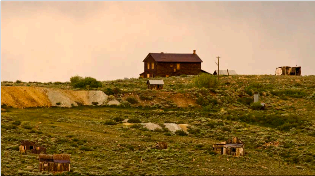
Bodie's railroad office, usually off limits to visitors, is now a stop on the Vista Tour.
