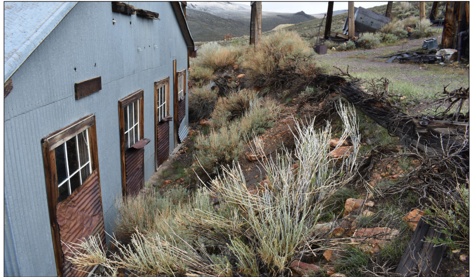
Bodie Foundation has launched a new fundraising project for the Stamp Mill. Work has started on erosion at the back of the building.
